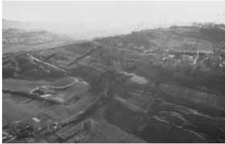
Figure 5.6 - Aerial view of the December 1982 Ancona landslide.
