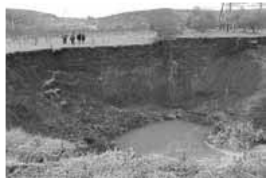
Figure 3 - Marcellina sinkhole (A. Colombi)
