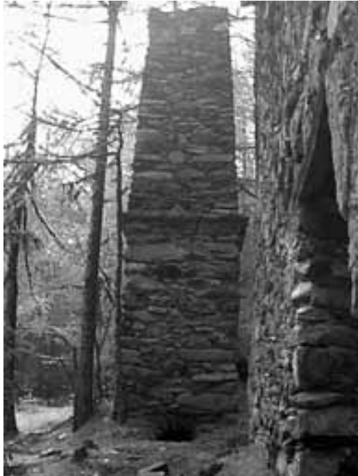
Figure 21 - Remains of the old foundry at Treves: a furnace structure.
