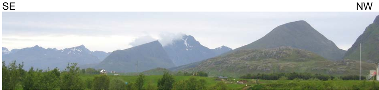
Fig. 37: SE-dipping low-relief paleosurfaces bounded by presumed steep fault escarpments resembling tilted and rotated fault blocks in the central Lofoten area, north of Leknes.
