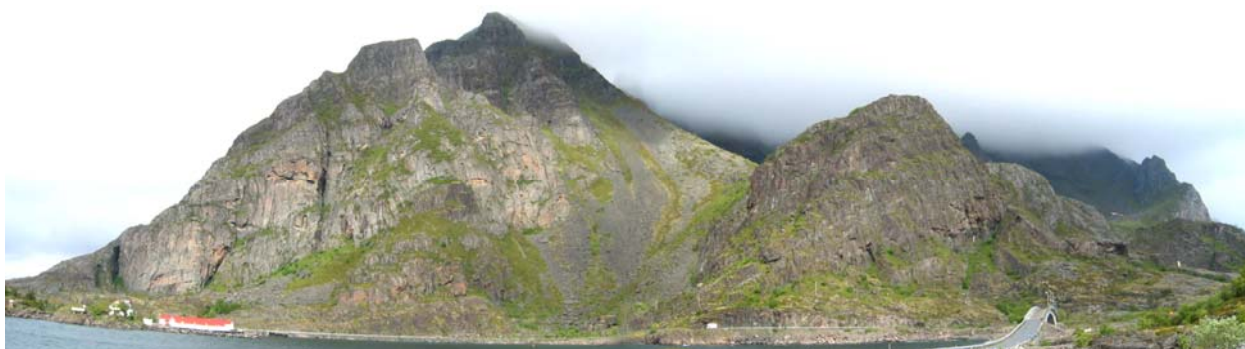
Fig. 43: Panorama view of the cliffs north of Henningsvær (bridge in foreground). Note gently W-dipping magmatic layering in the mangeritic rocks.
