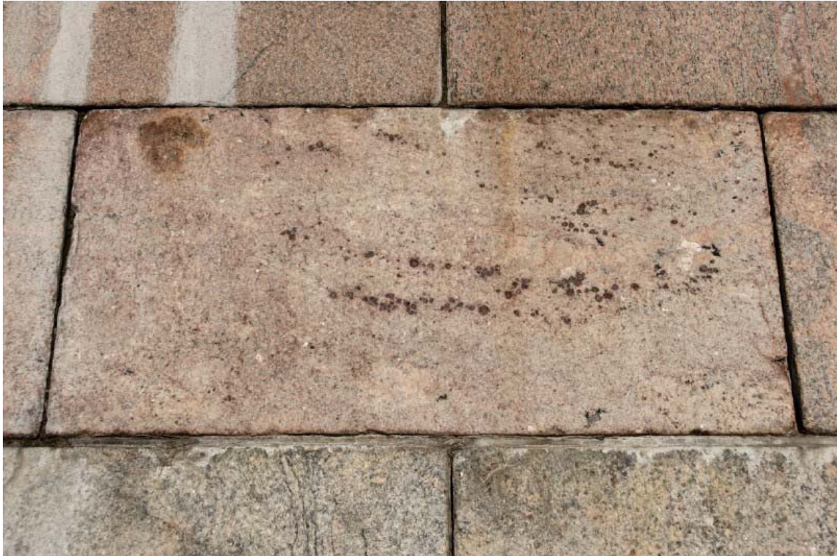
Figure 1. Garnet rich veins (remnants) in a granitic block (ca. 60 cm x 120 cm). Grounds of the Helsinki Cathedral. (N=6674964; E=3386495) Photo: Jukka I. Lehtinen.
