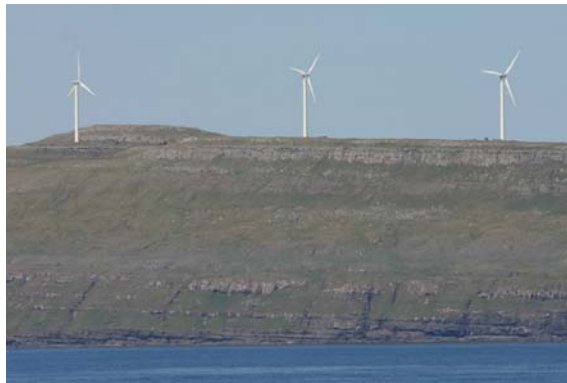
Fig. 128. View of the wind turbines built on lava flows of the Enni Formation, Neshagi, Eysturoy.
