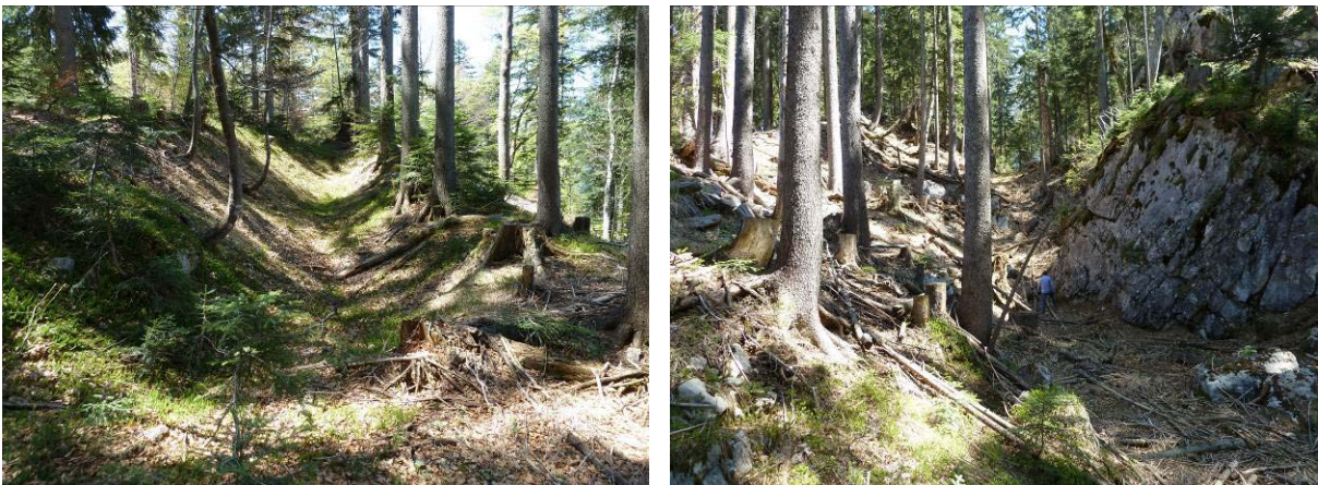
Figure 15. Signs of deep-seated gravitational slope deformation (minor scarps, transverse cracks and ridges) within the head of the Reppwand landslide.
