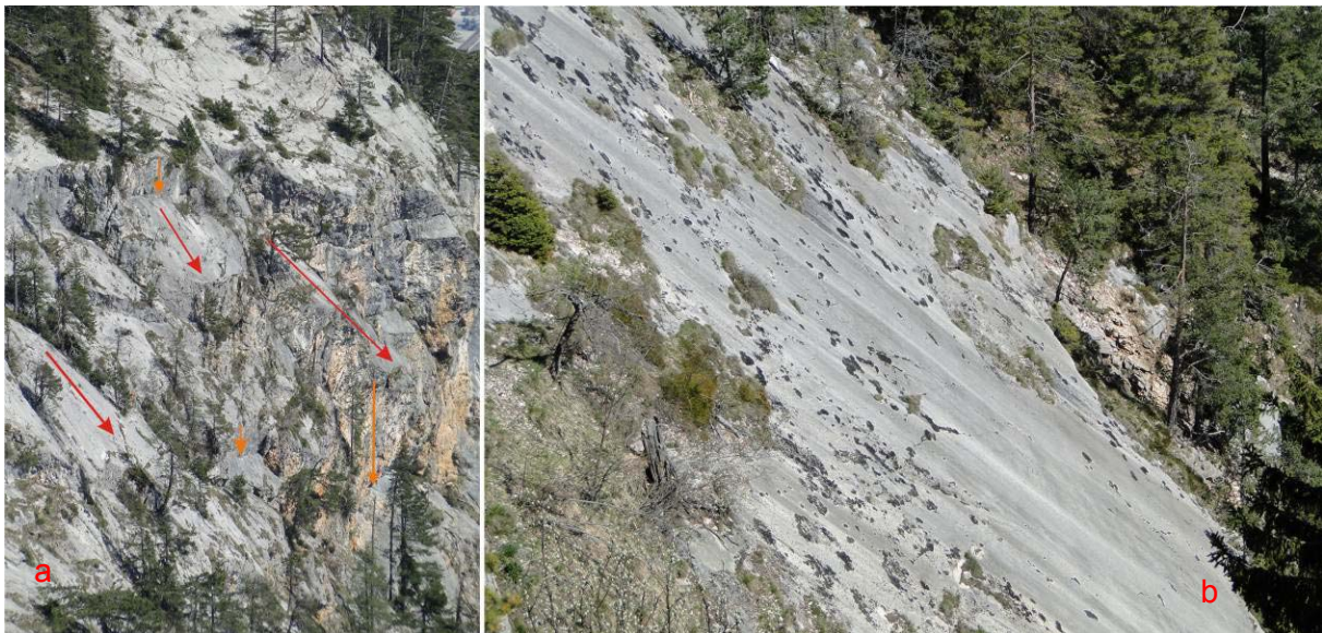
Figure 8: Outcrop on western part of the “Rote Wand”. (a) The different discontinuities: red colours show the dominant joint plane; (b) A view of the side plane, which is steeply inclined towards the south.
