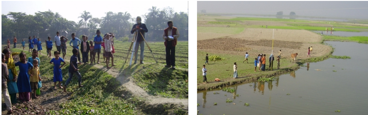
Figure 20 Leveling of irrigation wells at Titas/Daudkandi, pictures shot at the 11 th of December 2007
