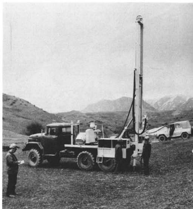
Figure 5: Drilling for groundwater in Central Asia.
