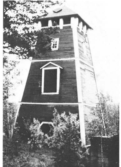
Old head frame at site of well-known former Orijarvi Pb-Zn mine, Finland. (Photo courtesy D.F. Sangster)
