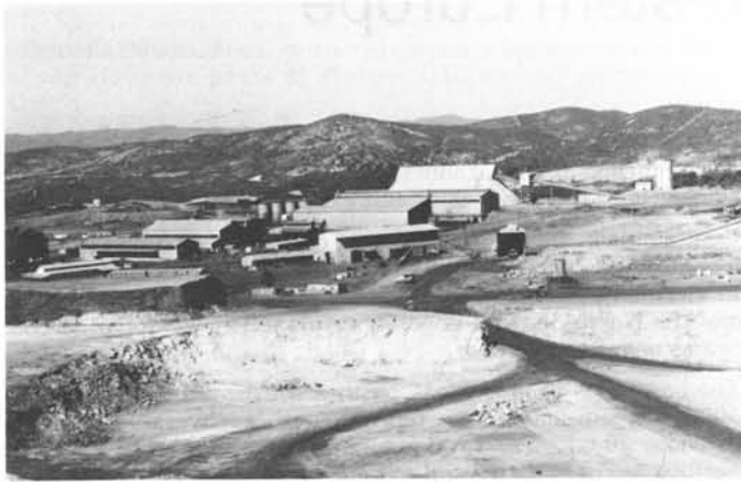
View to north of Cerro Colorado pit and mineral processing plant, Rio Tinto, Spain. (Photo courtesy R.V. Kirkham)
