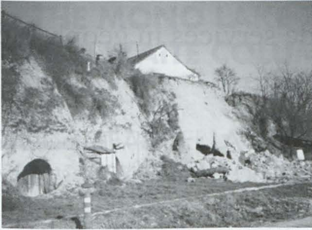
Fig. 3. Wine cellars mined in loess slope. Bátaszék-Lajvérpuszta, Tolna county.
