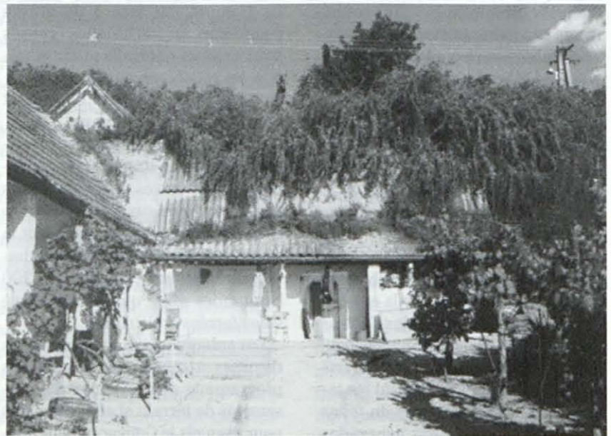
Fig. 2. An active cellar home in loess and the attached new house. Above a new level of houses and street, Ozora, Tolna county.
