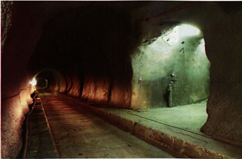
Fig. 1: View of the Mont Terri reconnaissance gallery (left) and one of eight niches (right) which have been excavated for the project. The tunnel walls are covered with shotcrete.
