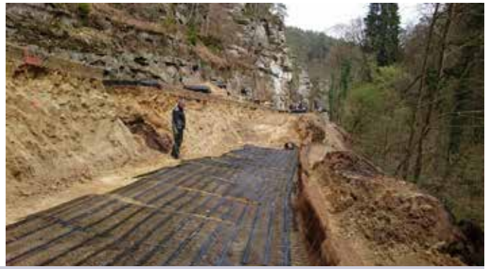
a b Figure 6: The TensarTech GreenSlope system: its principle (a) [reproduced with the permission of Tensar] and on site (b).
