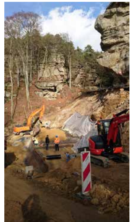
Figure 11: Stabilisation system under construction.
