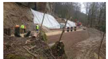
Figure 12: Rock outcrop integrated into the stabilisation system.
