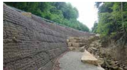
Figure 8: Stabilisation system under construction.
