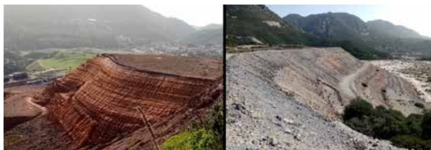
Figure 6: Extractive Waste Facilities. On the left Monteponi Mine red muds, on the right Masua Mine tailings pond.
