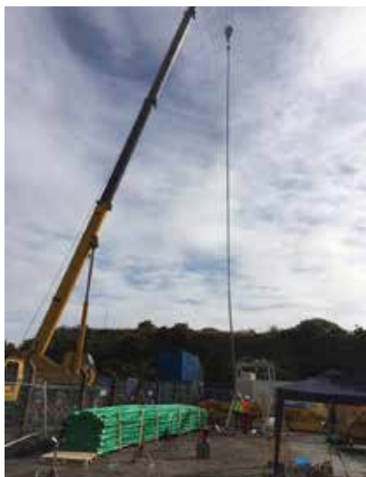
Figure 5: DGSW pipework being installed at the trial site.
