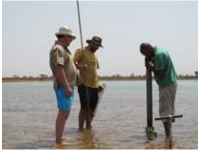
Figure 10: Hand-held drilling taking place on the banks of Niger. Kirina, Mali.
