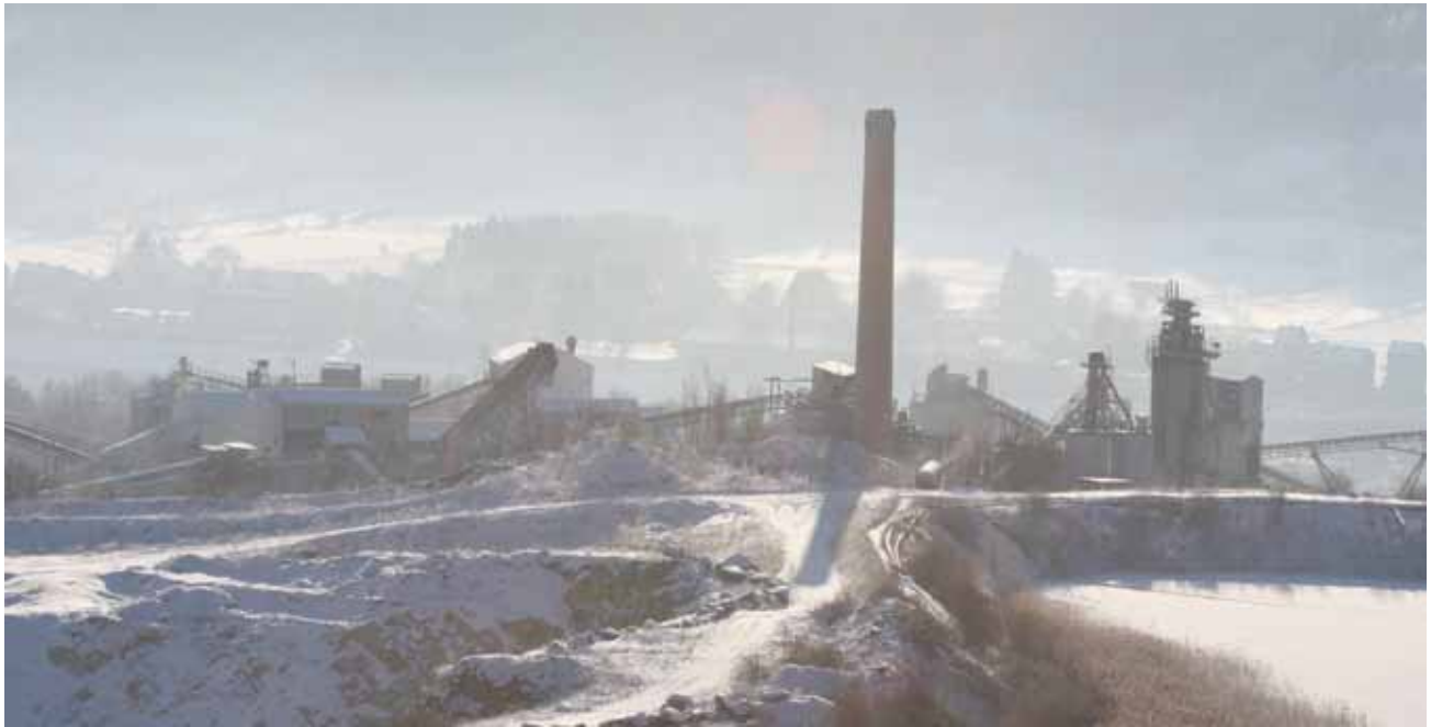
Figure 6: Overview during the wintertime of the Seilles (Andenne) quarry and plants services. (Goemaere, 2010b) (Photo: P. Timmermans).
