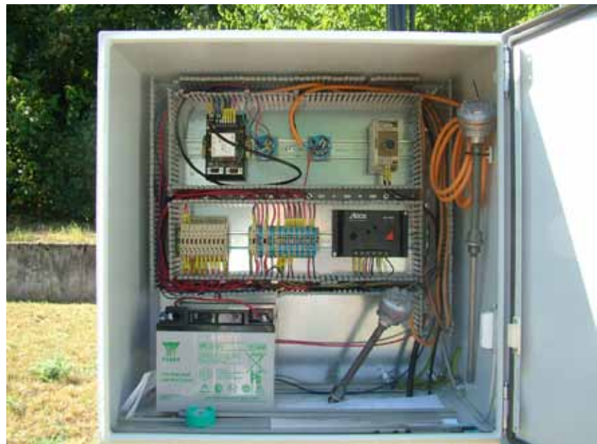
Figure 3: Mobile GSM/GPRS communication tester equipment.
