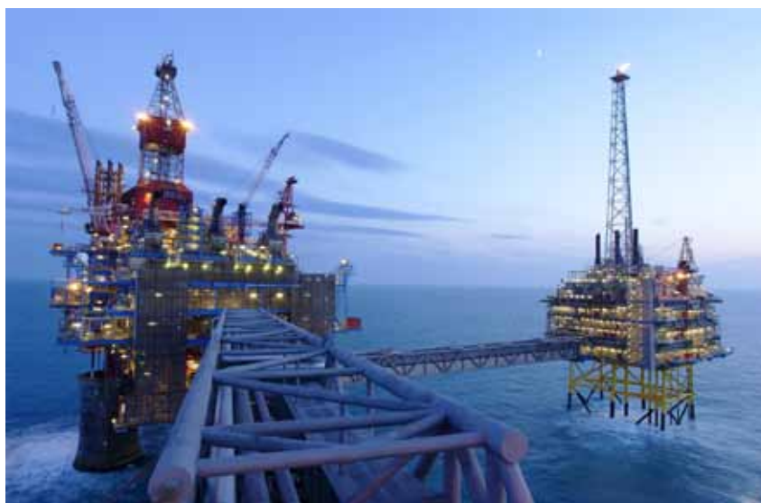
Figure 1: At the Sleipner project, natural gas is produced which is too rich in CO 2 to be marketed. Therefore about 1Mt of CO 2 is removed annually. Instead of releasing this CO 2 into the atmosphere, which is the standard practice, it is injected into an aquifer above the natural gas field (Courtesy Statoil).
