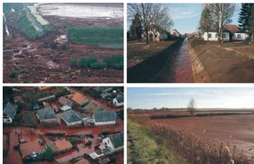
Figure 2. Impact of the red mud spill (Upper left: the breached dam as the contamination source. Upper right: the Torna Creek and its floodplain as the contamination pathway. Lower left: flooded village downstream as the human receptor. Lower right: flooded agricultural land as ecosystem receptor)
