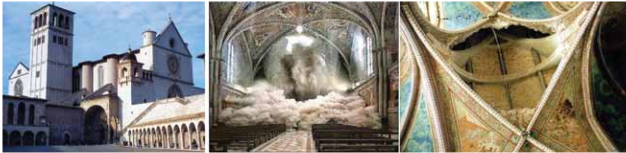
Figure 1. St. Francis Church in Assisi and the damage produced by the September 26, 1997 earthquake ( www.raffer.it ; www.archeomolise.it ; www.hotelfratesole.com )
