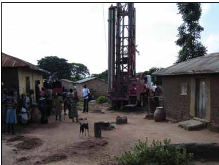
Drilling operations in Yava village
