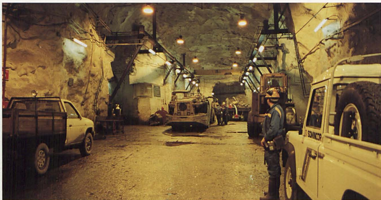
Neves-Corvo. Underground workshop.
