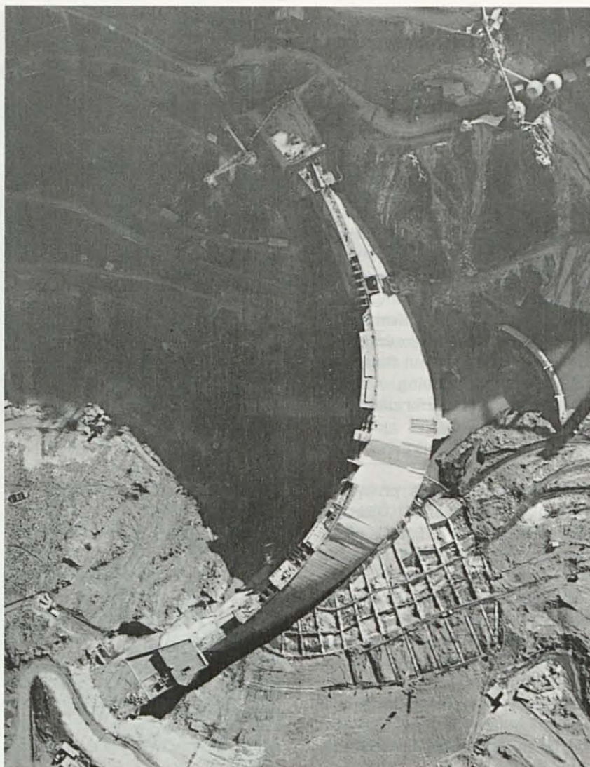
Aerial view of an arc dam.
