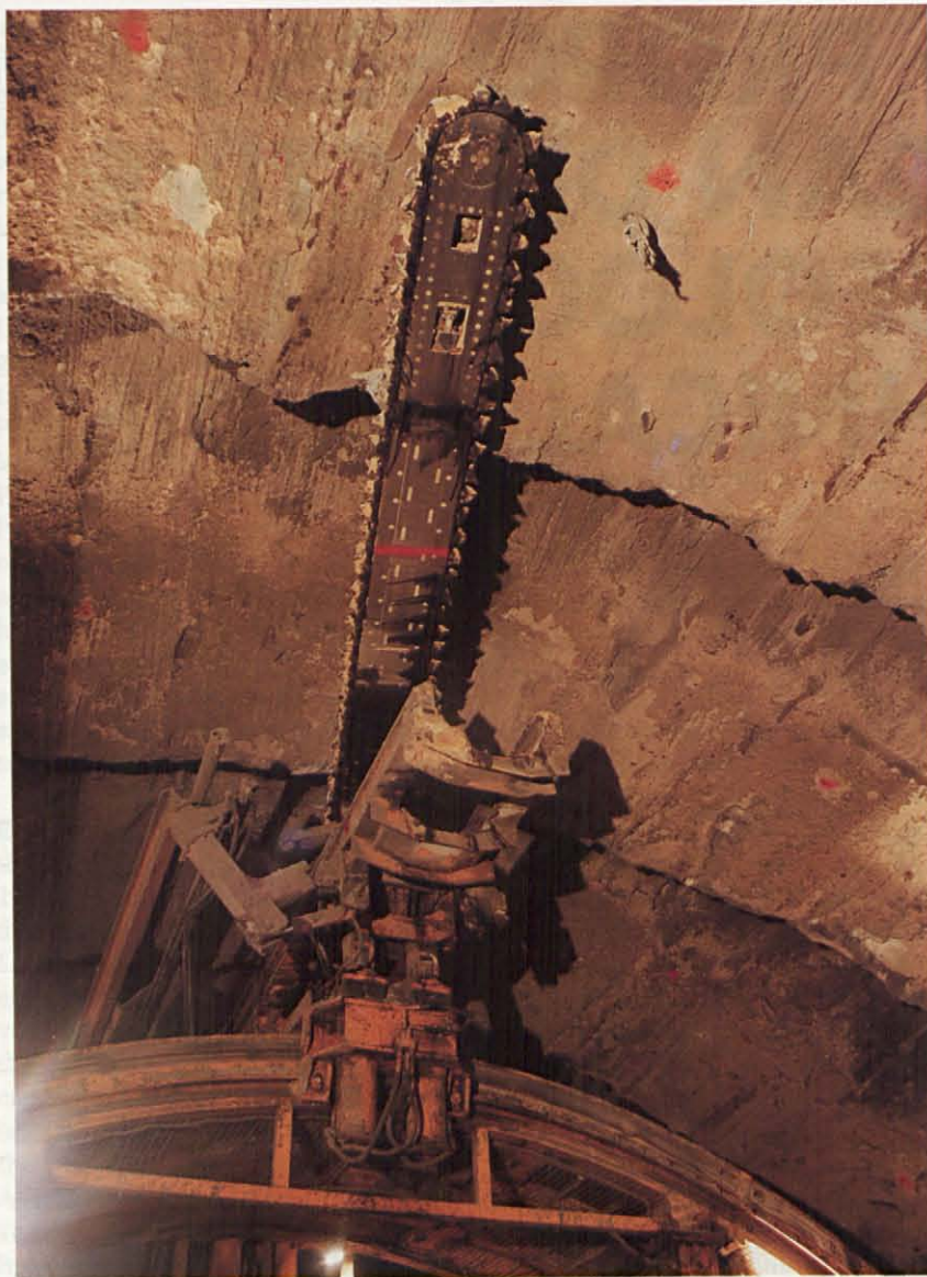
Mechanical precut machine. Detail of cutting saw Tunnels under El Pardo mountain. Madrid. (Spain).
