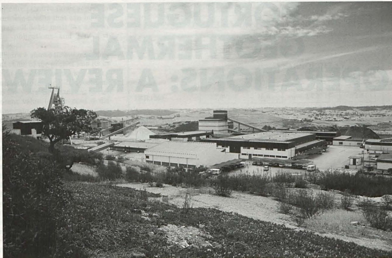
Neves-Corvo general view of the facilities.
