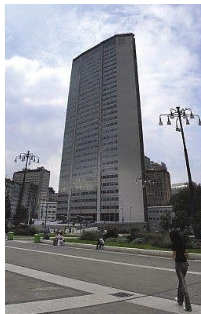
Milan (Lombardy): Pirellone skyscraper heating and cooling demand is covered by a ground source open loop system working since 1998
