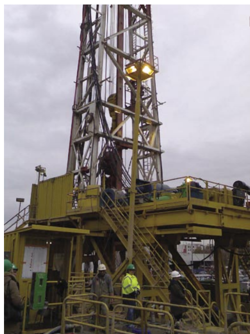
Figure 2. Geothermal drilling in the Paris Basin
