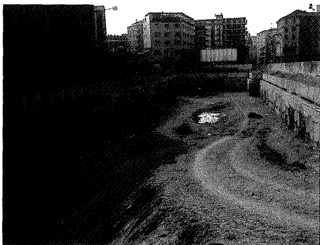
Figure 2. Diaphragm walls and tie rods, site of Bacchiglione
