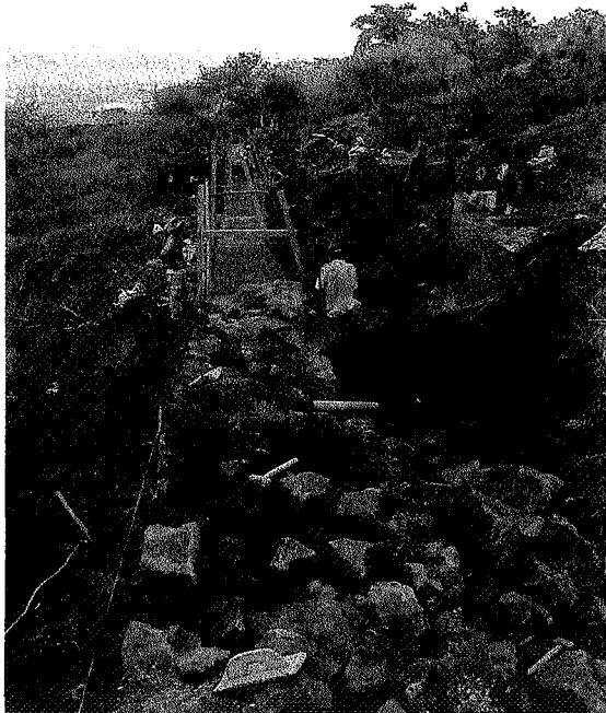
Building of retention wall, southern San Miguel volcano slope, El Salvador, 2002
