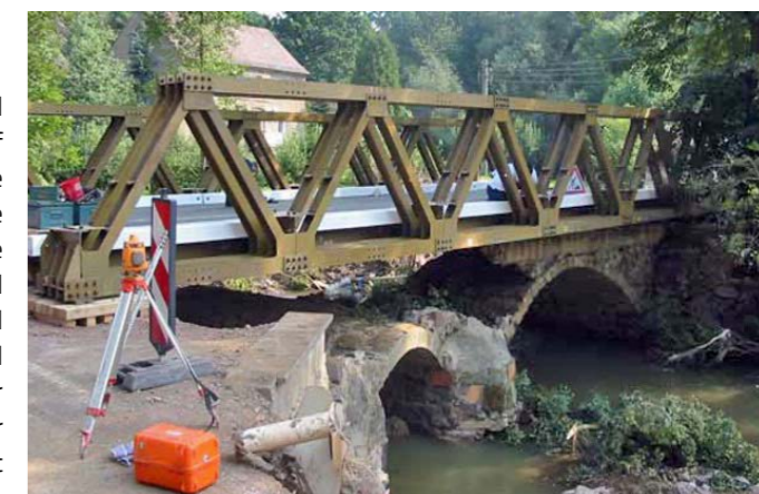
Figure 1. Bridge destroyed in a flood, mobile overpass erected by THW (photo by THW OV Fürth)
