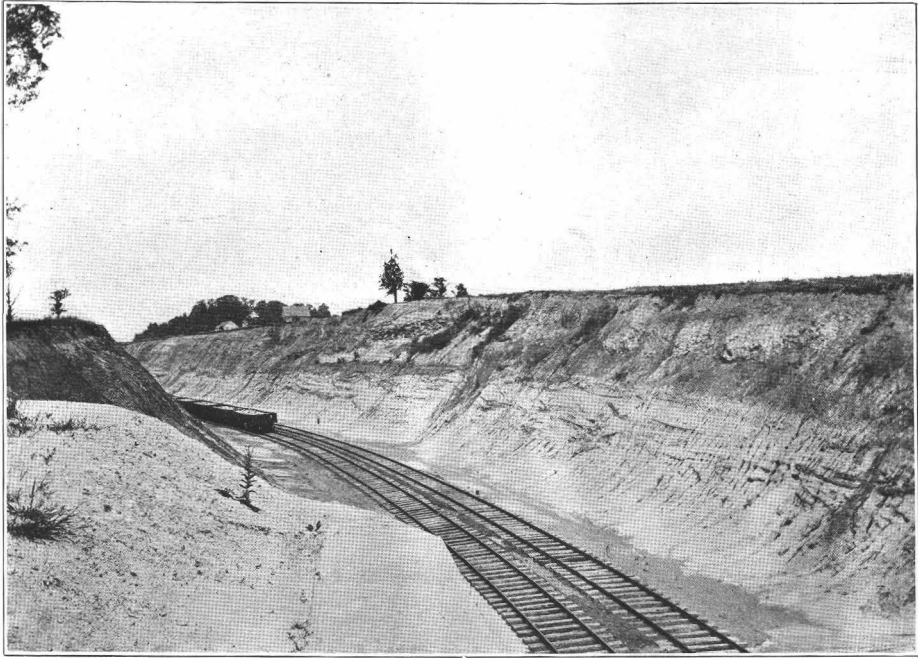
FIGURE 1.—BELT LINE (BALTIMORE AND OHIO RAILROAD) CUT, BALTIMORE CITY Showing Characteristic Sands and Gravels
