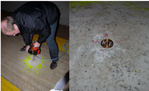
Figure 1: overview of the geodetic network and mounting of benchmarks
