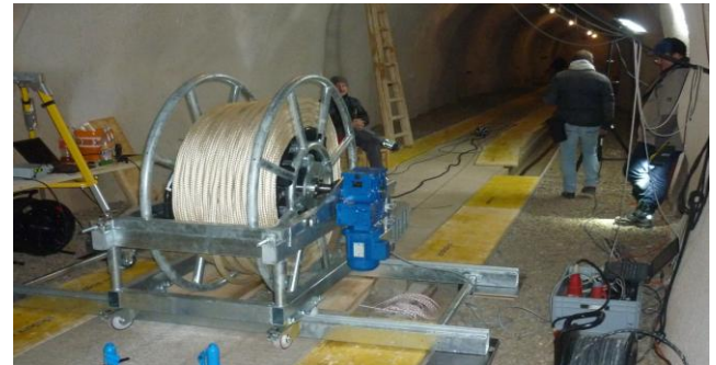
Figure 2: The winch system with LCP encased sensor cable shortly before lowering the sensor.
