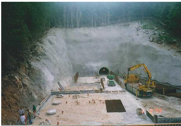
Figure 1: Conrad Observatory building fundament construction (credit: Wilhelm)
