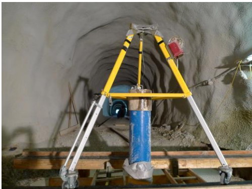
Figure 1: Borehole with casing.
