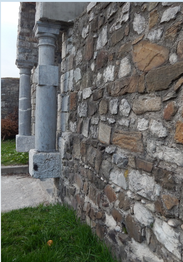
Figure 1: Several types of natural stones are used for architecture elements in cultural heritage; here, the restored Roman wall in Ljubljana.
