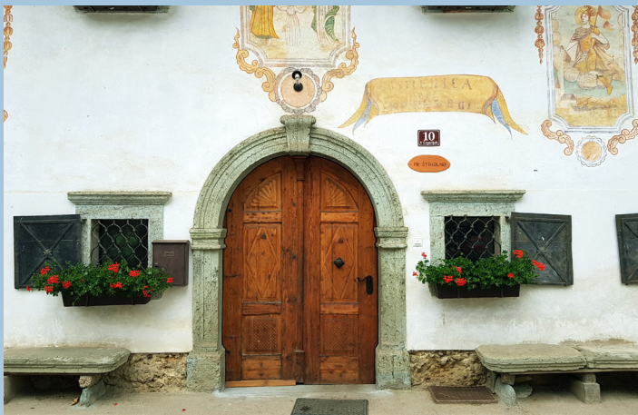
Figure 4: Country house in Zgornja Besnica with entrance portal, window frames, and benches made of green Peračica tuff.
