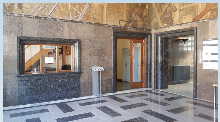
Figure 2: Different Cretaceous limestones with rudist shells in the lobby of the Montanistika building (1937) in Ljubljana. The dark Kazlje limestone and the light grey Kopriva limestone are from Slovenian Kras, while the brownish one is from the island of Brač, in Croatia.
