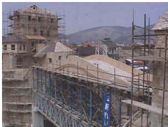
Fig. 2. The bridge under reconstruction
