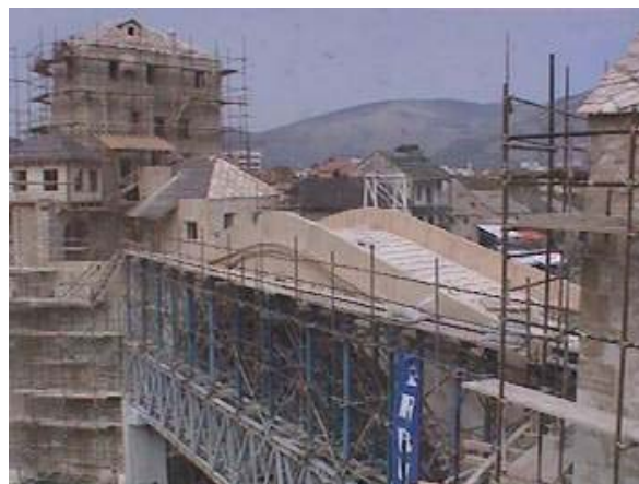
Fig. 2. The bridge under reconstruction
