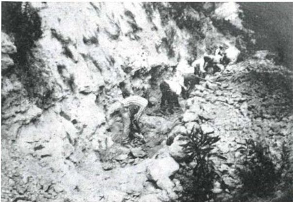
Figure 13: Excavation at Adrianos ravine (MTLA) in 1963 (photo reproduced from MELENTIS, 1968).
