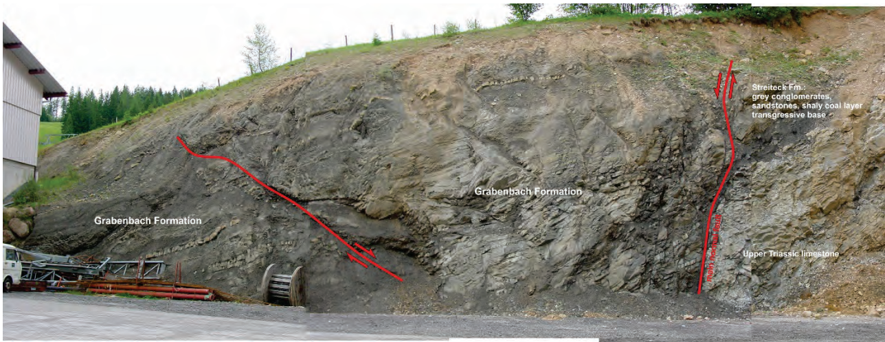
Text-Fig. 10: Rußbach, parking area at the cable car station (Hornspitzbahn). Basal Grabenbach Formation with ammonites and inoceramids, resting upon layers of shales with pebbles, coalseam, corals, gastropods (Streiteck Formation). Transgression upon Triassic rocks (right side).
