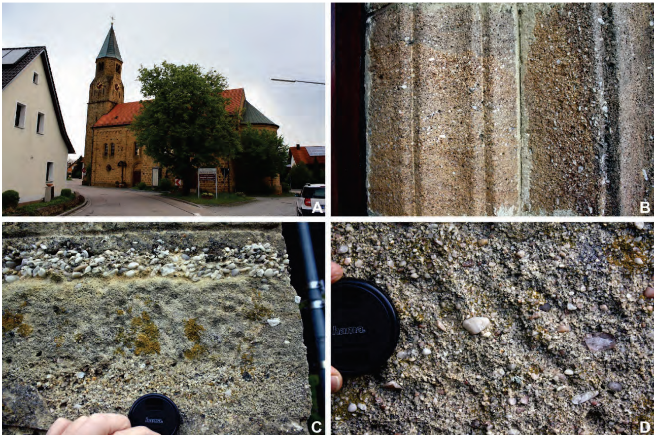
Text-Fig. 27: Freihöls Member of the Roding Formation (Middle to Upper Turonian) used as freestone at the parish church “Mariä Namen” in Neubäu am See. A: the church as seen from the south. B: door frame showing the immature, coarse-grained fabric (field of view ca. 1 m). C: better sorted facies consisting of dm-scale units grading from quartz (micro-)conglomerate to coarse-grained sandstone; note the good rounding of the quartz granules and pebbles in the upper bed (lens cap for scale). D: close-up view of the poorly sorted pebbly coarse-grained sandstone facies of the Freihöls Member (lens cap for scale).
