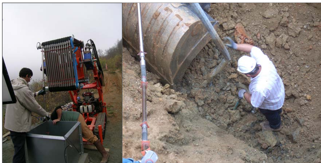
Fig 1, 2: DMS column installation (28 th October 2008) and removal (13 th July 2009) – Bagnaschino site.
