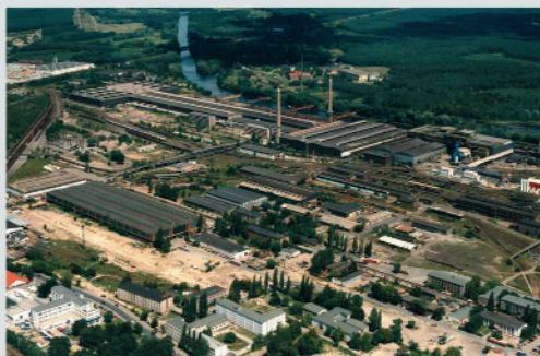
Areal view of the Hennigsdorf steel works and rolling mill
