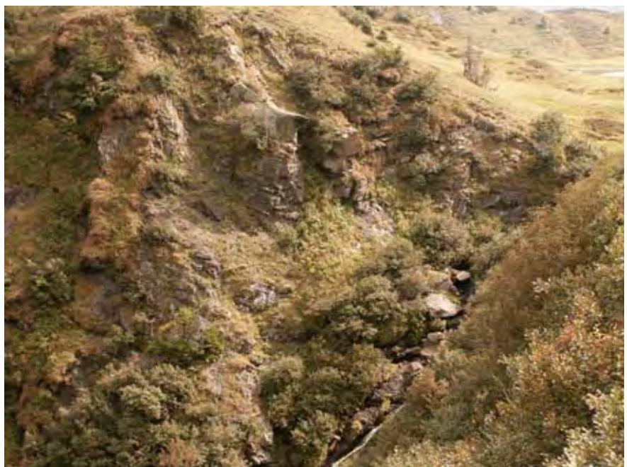
Fig. 13: Section on the right bank of the outflow of Lake Zollner with sketch-map.
