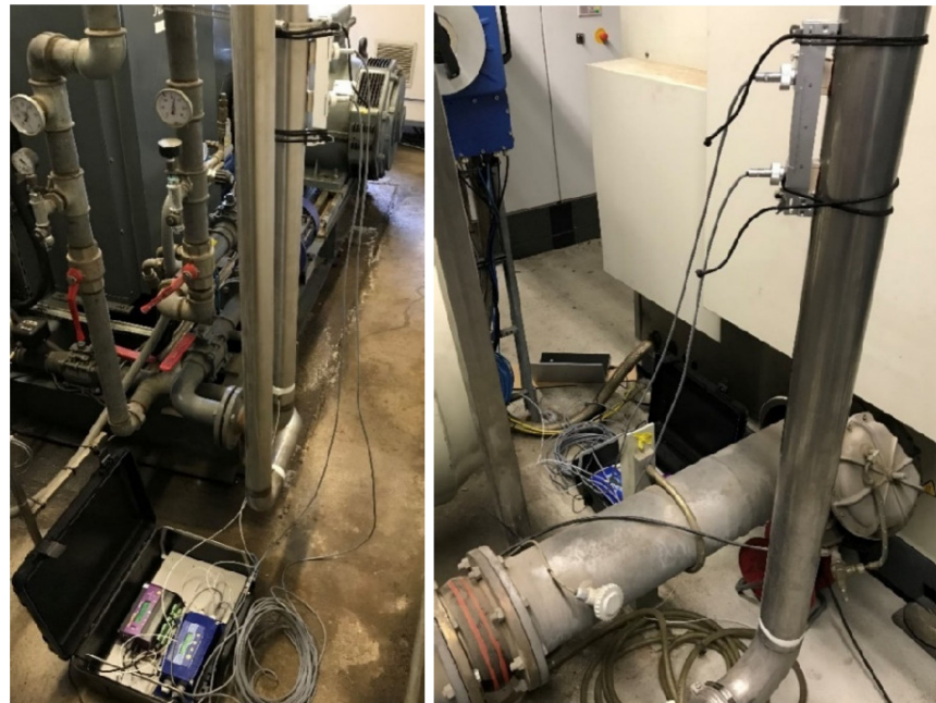
Figure 5. Measurements on the HDD systems: Atlas Copco (left)—LMF (right).
