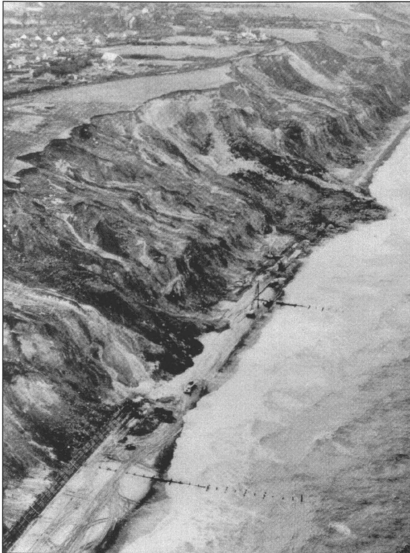
Fig. 27: Landslide in the vicinity of Sidstrand, Norfolk (acknowledgements to Aerofilm Ltd.).
