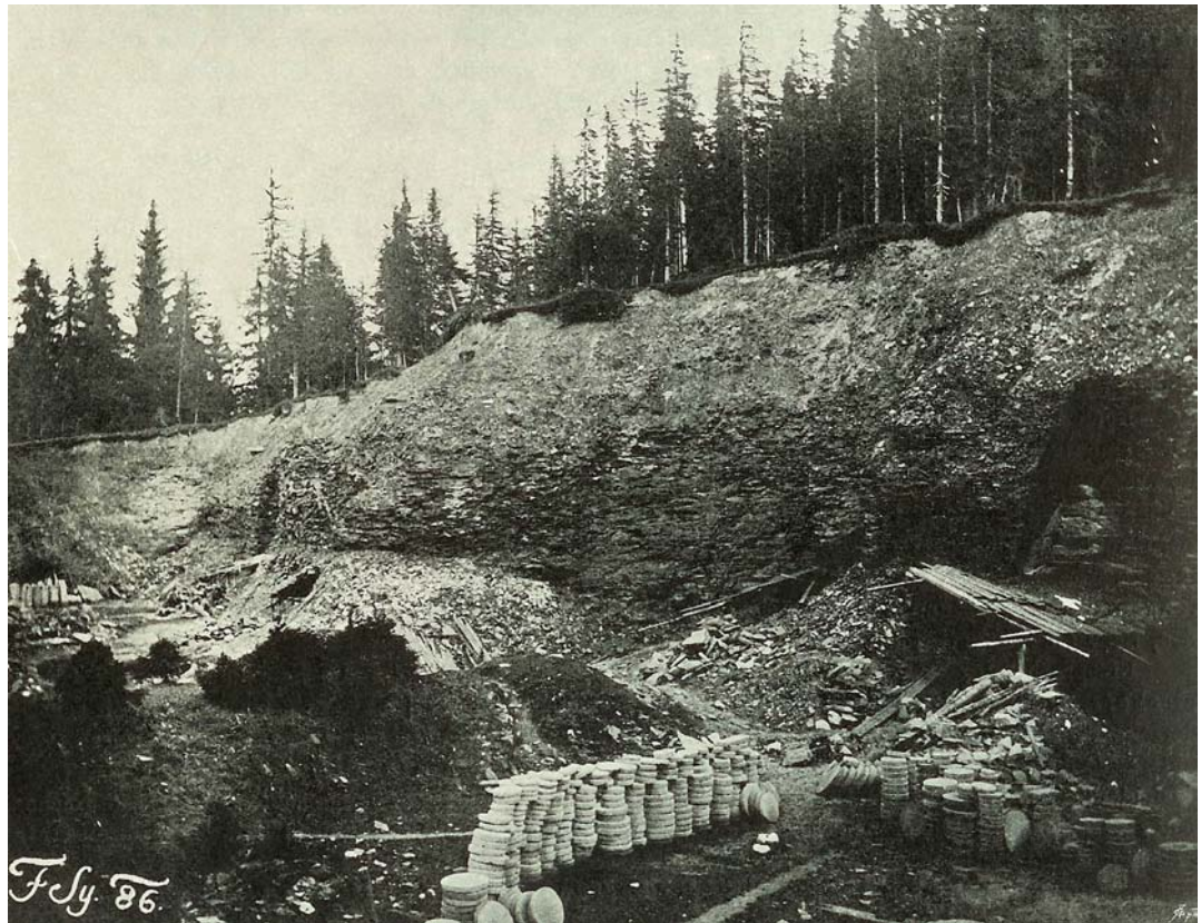
Text-Fig. 3. The photo by Friedrich Simony from the year 1886 shows one of the grindstone quarries (?or the only one at that time) in about 1300 m altitude. Grindstone products are prepared for the transport in the valley (Gosau, 736 m).
