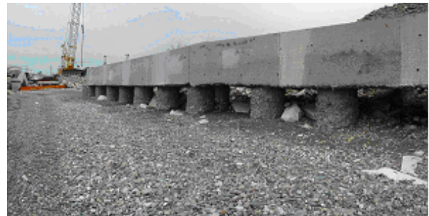
Figure 1 – In the background – the port under construction (March 2011).
