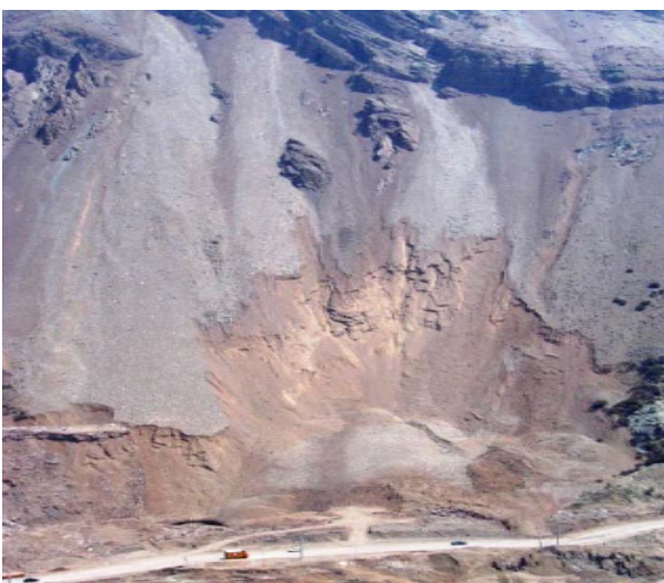
Figure 5 – A general view of third station.
