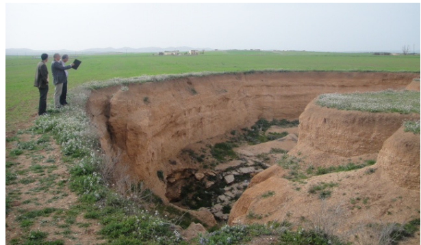
Fig.2, The first spectacular sinkhole in Douamis locality.
