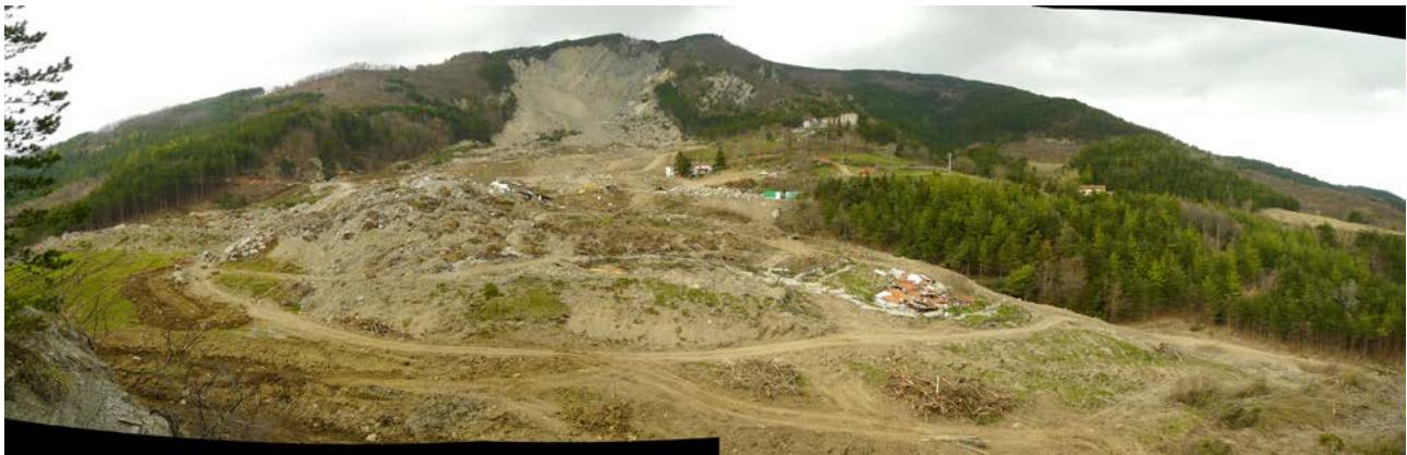
Fig. 1 – Panoramic view of the landslide area on 2010 march 27 th .
