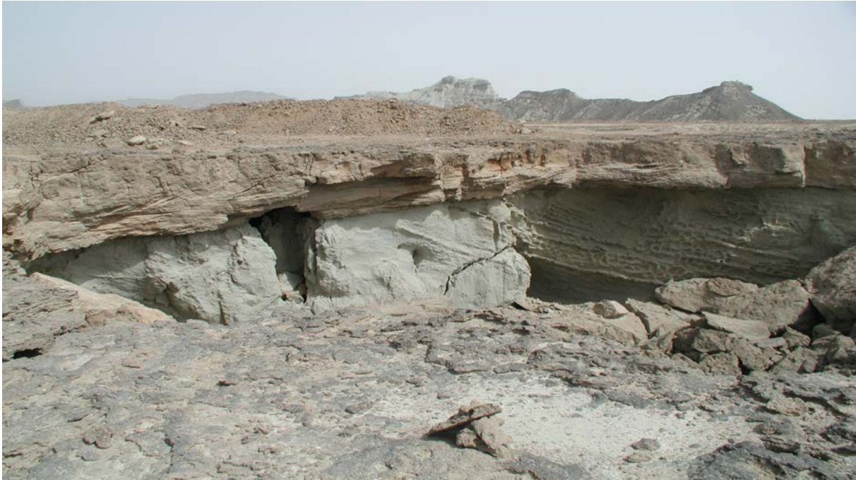
Figure 1- The subsurface erosion, which led to sloughing and bank failures.
