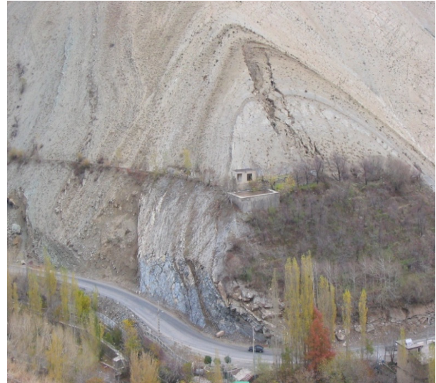
Figure 6 – A general view of station 4 (Maygon area).
