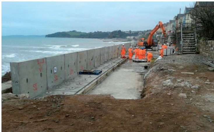
Figure 3. Constructions erection aiming at high water protection
