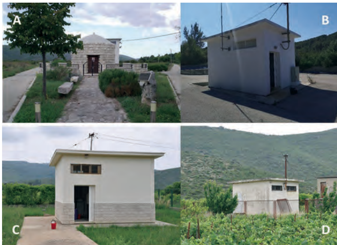
Figure 1. Public water supply wells in Blatsko Polje. A – Studenac, B – Gugić, C – Prbako, D – Franulović-Prcalo
