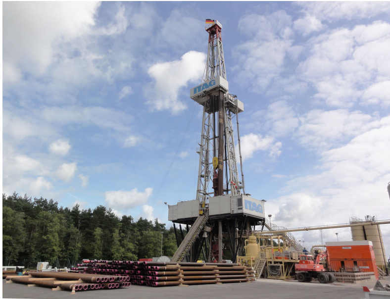
Figure 46: Conventional drilling rig at the geothermal project in St. Gallen 16 .
