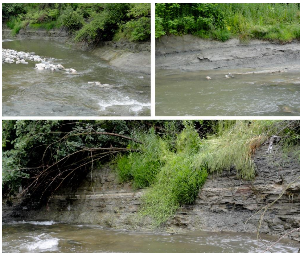
Fig. 4.3.1. The Valjevo Formation. The three different images of the Ribnica river shoreline with exposed the massive silty clay and silts (bottom part, above) and more laminated chalk and marl (above, right and below).
